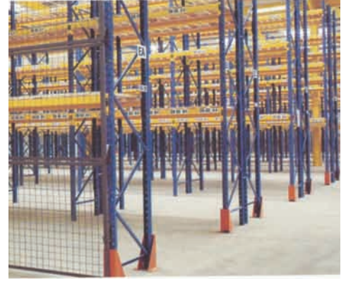
Column guards and mesh screens.
